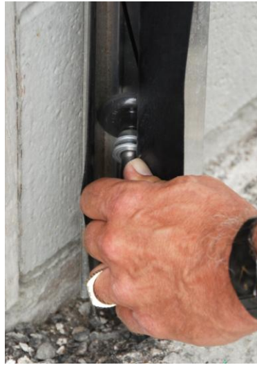
Photo #2 (Removing Rollers From Extrusion)
