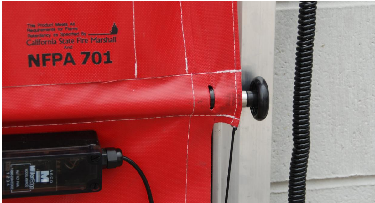
Photo #4 (Roller Fully Inserted In Pulltrusion)
