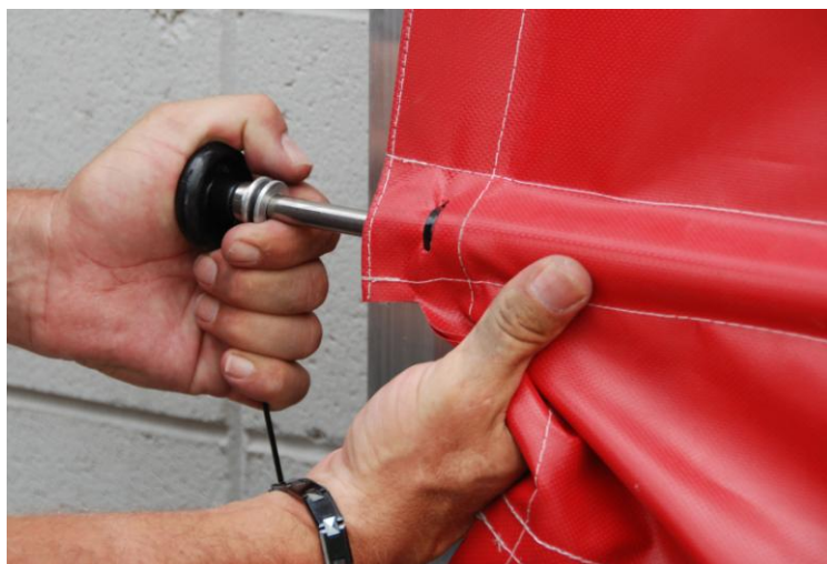
Photo #3 (Inserting Roller Into Pulltrusion)
