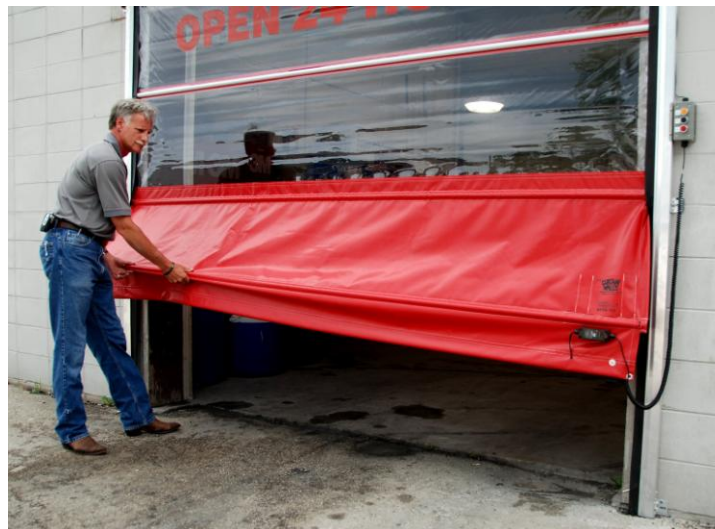
Photo #1 (Free Door Material From Opening)
